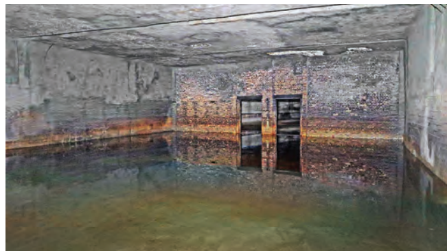
Dividing wall in Tiergarten tunnel. Photo Clive Penfold
